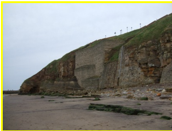
Natural cliff protected with block/brickwork (Asset Refs. 1221D901D0802C09)
