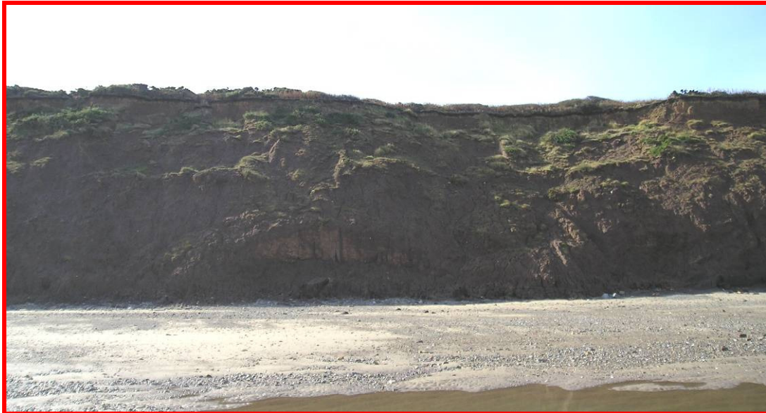
MU29/BH Headscarp recession and slumping of material onto the beach (Totally Active)
