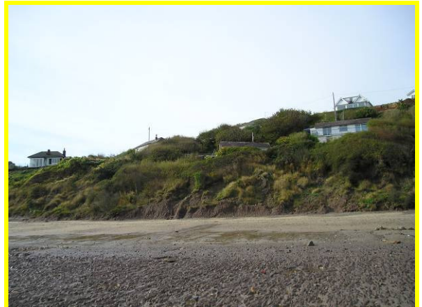
MU29/AR Toe erosion at Flat Cliff (Locally Active)
