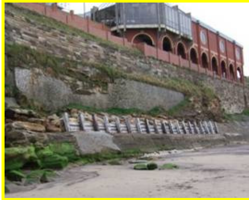
Overview of assets (Asset Refs. 1221D901D0802C05 and C15)
