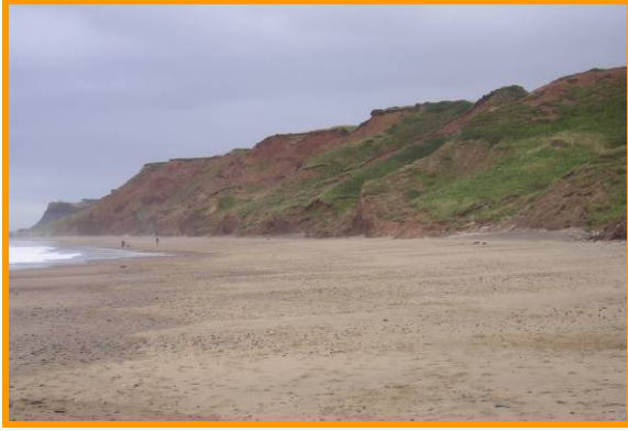
MU10/2 The collapsing till cliffs at Upgang Beach (Partly Active)
