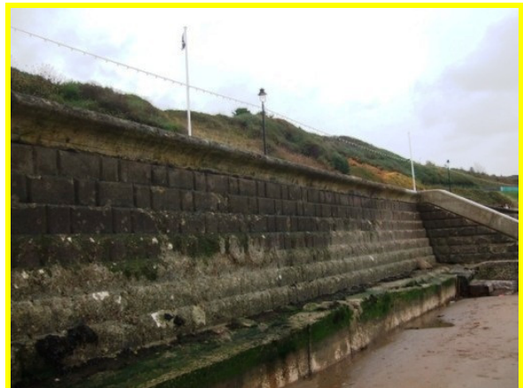
Exposed concrete toe (Asset Ref. 1221D901D1201C24)
