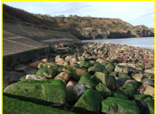
Concrete revetment located in the north of Sandsend (Asset Ref No.1221D901D0701C02)
