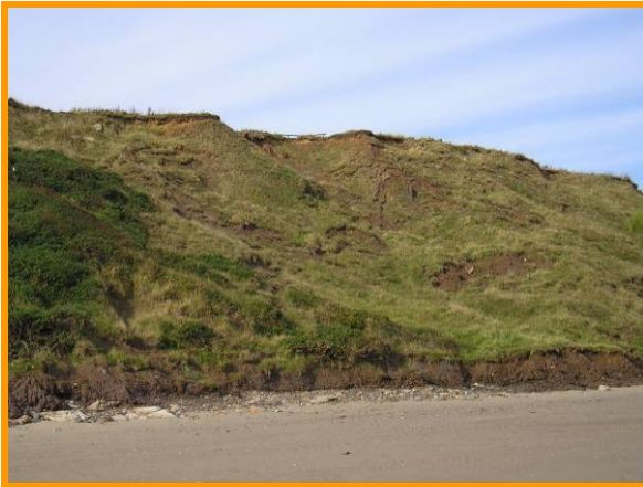
MU29/AO Intense erosion at the toe and headscarp, sliding mid-slope (Partly Active)
