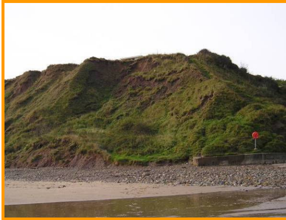
MU29/AJ Very common areas of intense erosion (Partly Active)
