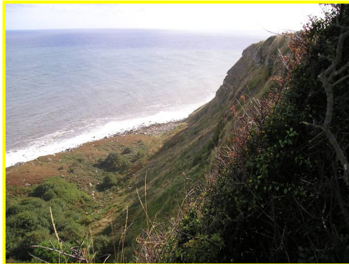
MU19/3 Showing localised erosion (Locally Active)
