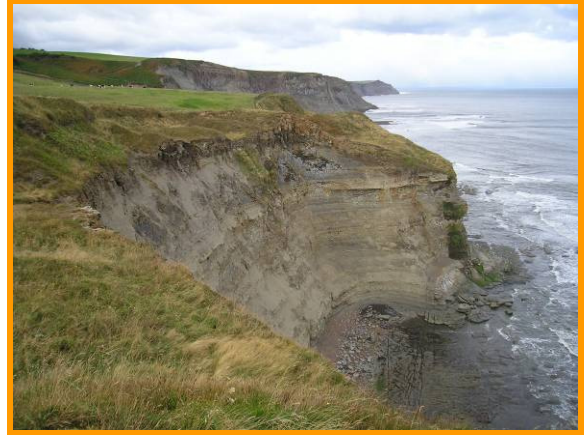
MU15/3 Ongoing erosion and evidence of small scale rockfall (Partly Active)
