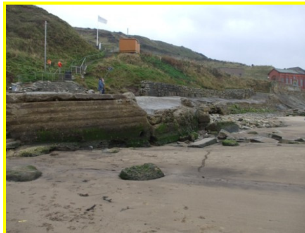
South end defence of the pumping station (Asset Ref. 1221D901D1402C06)
