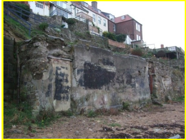
Wall at East side of harbour (Asset Ref. 1221D901D0803C09)
