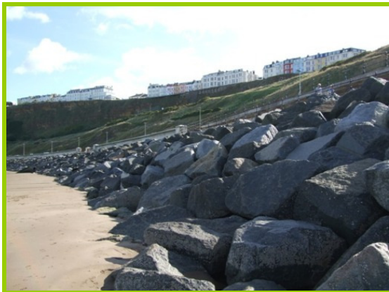
Overview of rock armour with raised crest wall (Asset Refs. 1221D901D1202C01)
