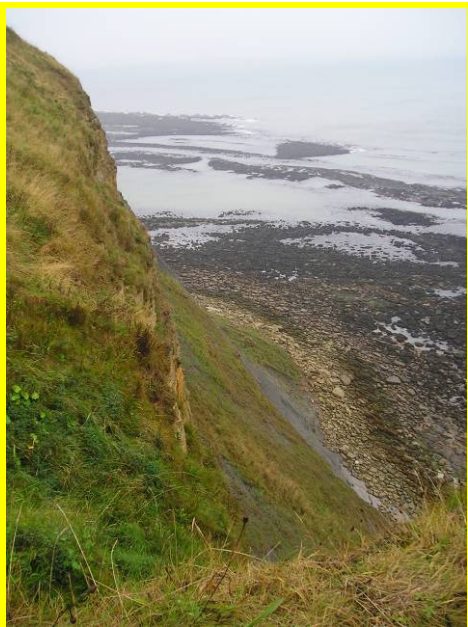
MU26/AF Rockfall evidence at the unit toe (Locally Active)
