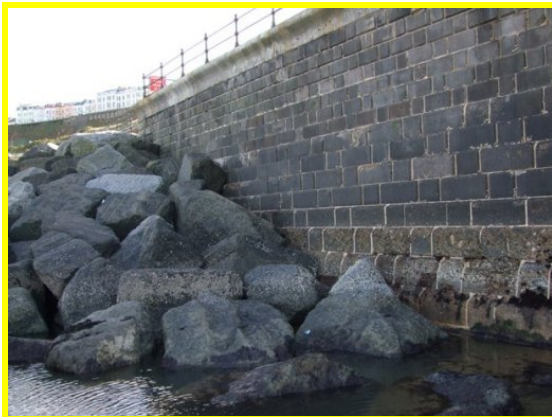
Overview of construction (Asset Ref. 1221D901D1202C23)
