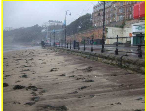
High beach level along sea wall running in front of Foreshore Road, South Bay (Asset Ref. 1221D901D1301C15)
