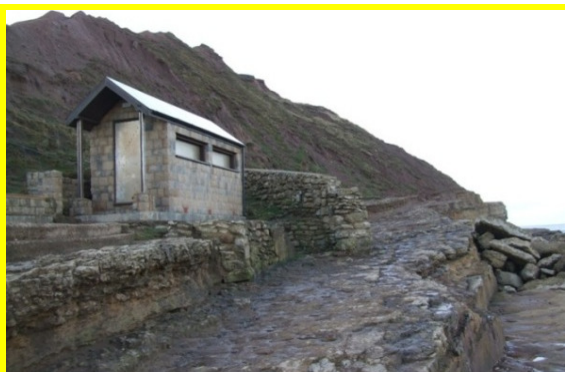
View of wall and cabin looking North West (Asset Ref. 1221D901D1502C01001)
