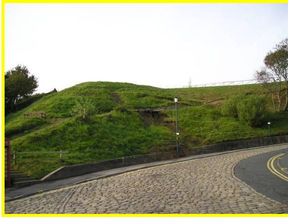
MU28/Z Recent landslide activity and footpath closure (Locally Active)
