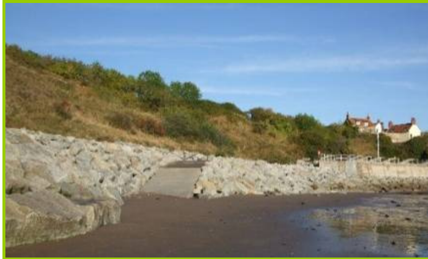
Looking northwards at the rock armour (Asset Ref. 1221D901D1003C07)
