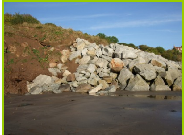
Extent of rock armour, showing 'end effect' (Asset Ref. 1221D901D1003C07)
