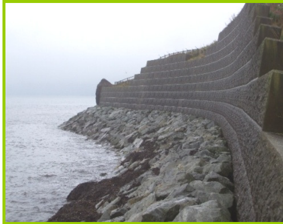
Sea wall at the northern end of Mu16A (Asset Ref. 1221D901D1003C01)
