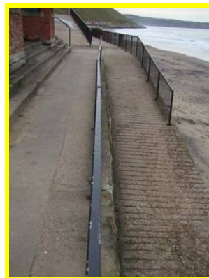
View of capping and promenade (Asset Ref. 1221D901D0802C06)
