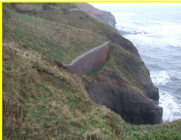
Brickwork wall at Deepgrove Wyke (Asset Ref. 1221D901D0603C01)
