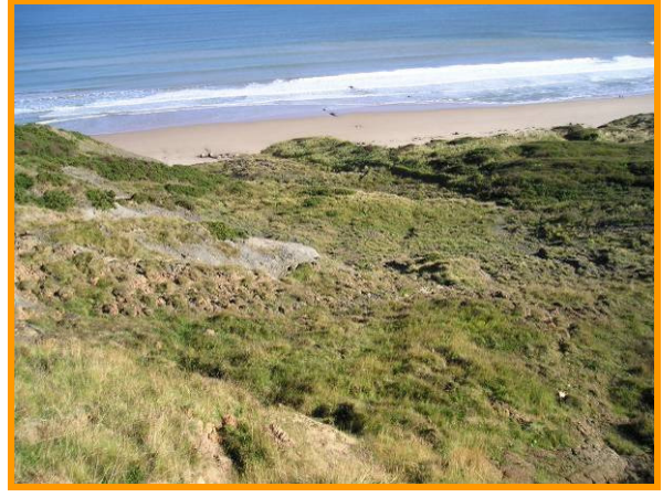
MU29/CD Mid-slope cracking and sliding (Partly Active)
