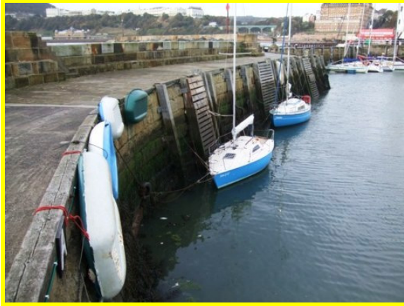
Overview of wall showing newer timber fenders (Asset Ref. 1221D901D1301C16)
