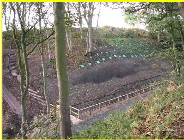
MU28/Z New slope stabilisation works to the ravine (Locally Active)
