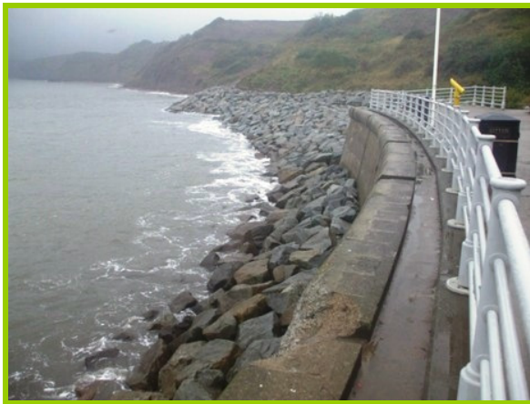
The rock armour, sea wall and promenade above (Asset Ref. 1221D901D1003C10)
