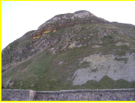
MU21/2 Well jointed hard rock layer within this unit (Locally Active)
