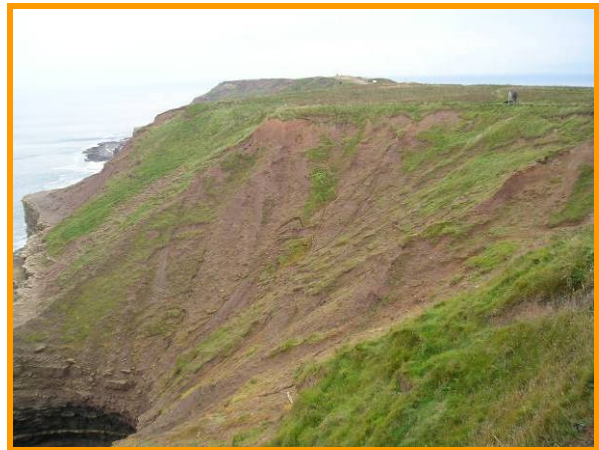
MU27/BC Slumping, sliding and rilling (Partly Active)
