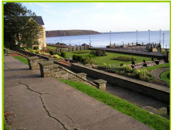
MU28/Y Repaired cracks to footpath (Inactive)
