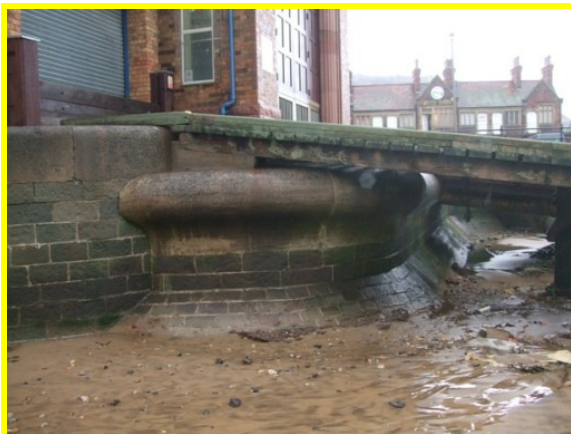
View of blockwork wall beneath life boat station (Asset Ref. 1221D901D1301C08)
