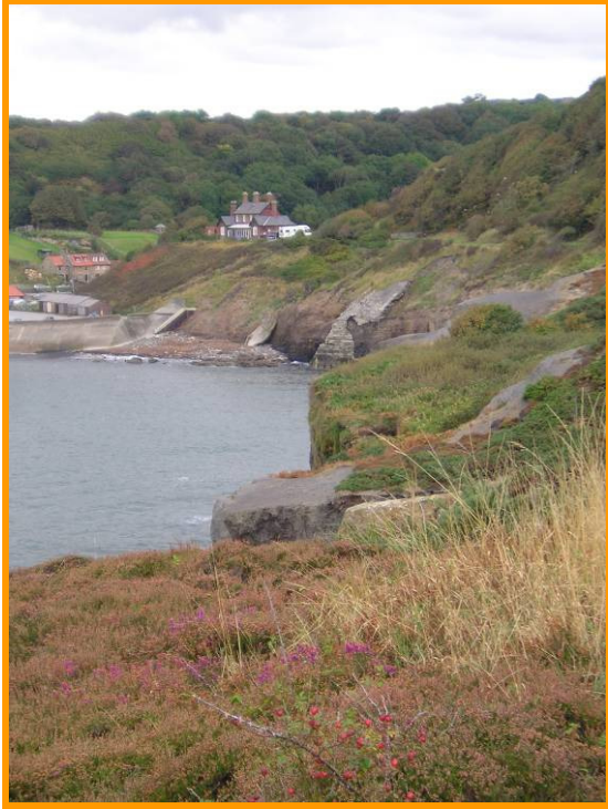
MU8/15 Erosion just north of Sandsend (Partly Active)
