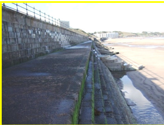
Looking north along berm from south end (Asset Ref. 1221D901D1201C08)
