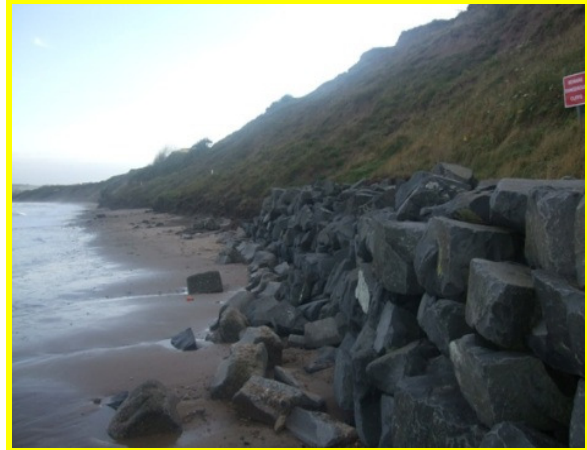
Rock revetment with gabion baskets beneath (Asset Ref. 1221D901D1602C02)
