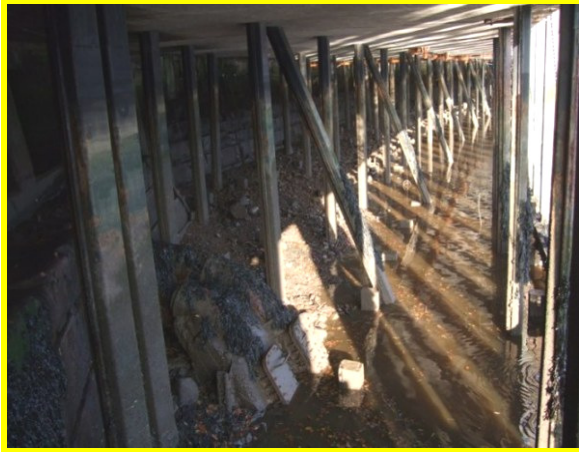
Concrete extension of promenade supports (Asset Ref. 1221D901D0803C06)
