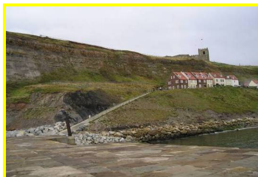
MU12/1 Localised erosion at the toe and headscarp (Locally Active)
