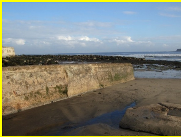
Overview of breakwater (Asset Ref. 1221D901D0601C02)
