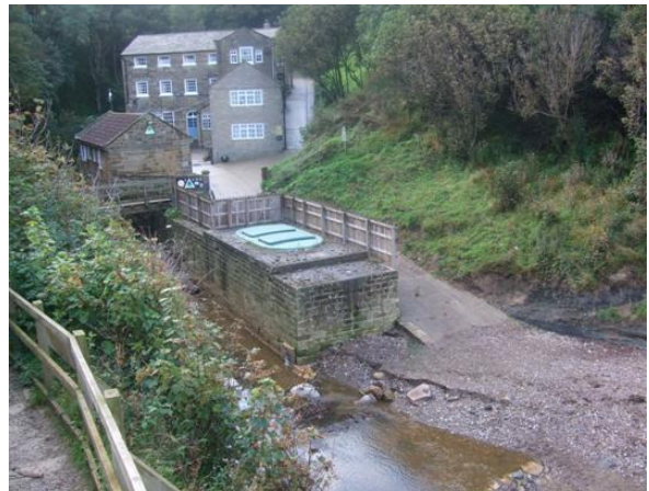
Looking upstream at Boggle Hole Youth Hostel, footbridge, slipway and fuel bund.
