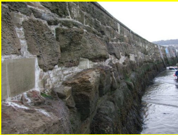
Filled and repaired wall (Asset Ref. 1221D901D1301C16)
