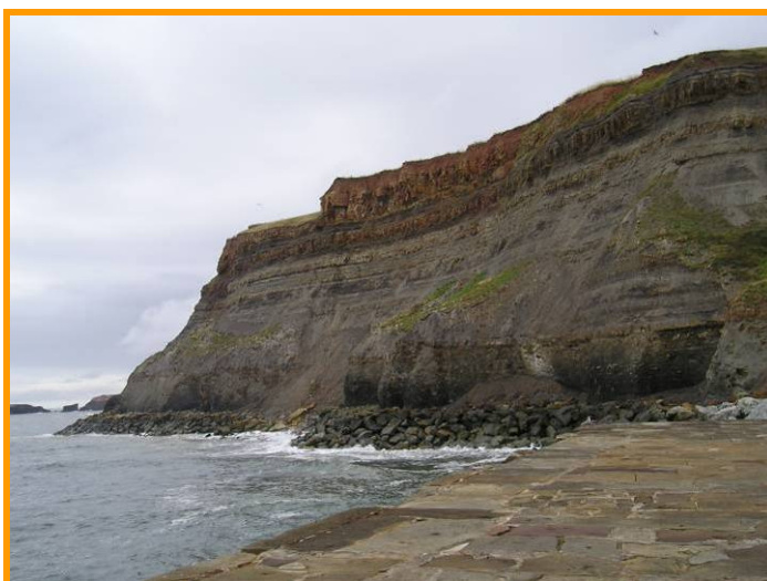
MU12/2 Looking east from Whitby's East Pier showing recent failure from the cliff top (Partly Active)
