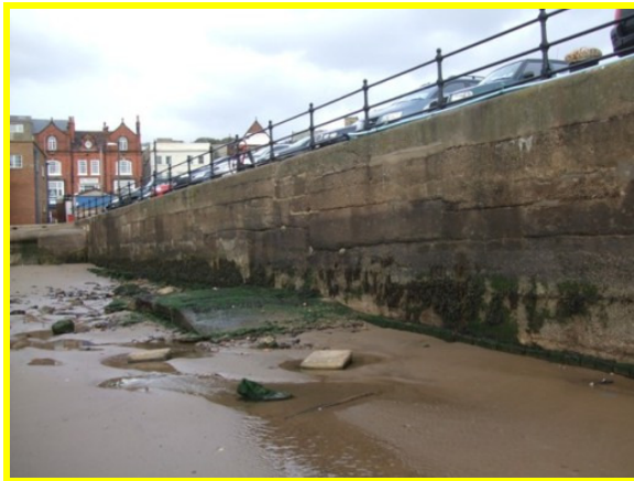
Overview of wall (Asset Ref. 1221D901D1301C19)
