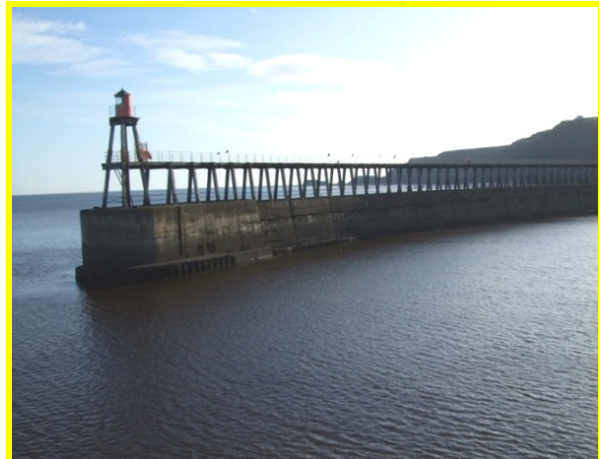
East breakwater (Asset Ref. 1221D901D0803C04)
