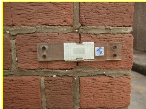
Tell tale on wall of life boat station (Asset Ref. 1221D901D1301C08)
