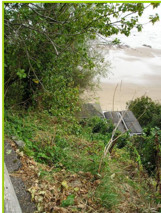
MU22/3 Looking down towards the cliff lift (Inactive)
