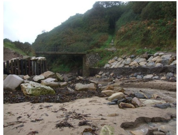
Rock armour revetment at the mouth of Stoupe Beck (Asset Ref No.1221D901D1003C08)
