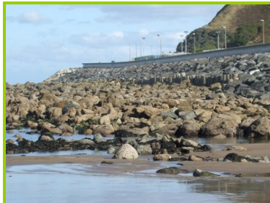
Overview of rock armour with concrete piles visible (Asset Refs. 1221D901D1202C03)
