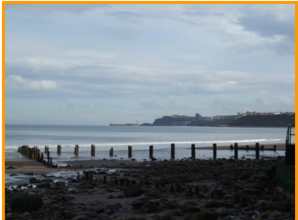
Timber groynes in front of Sandsend (Asset Ref. 1221D901D0702C01)
