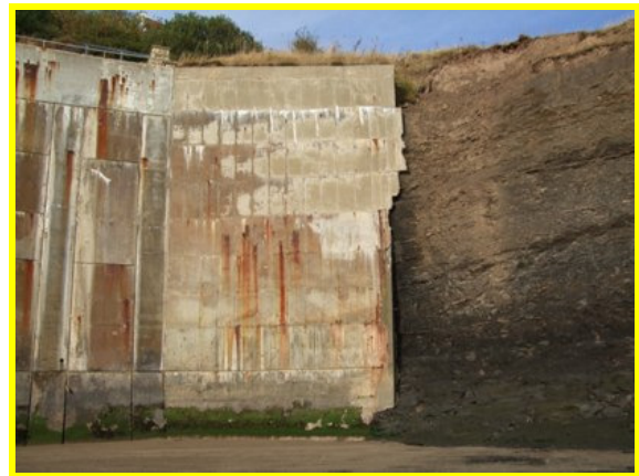
Joint between defended and undefended section (Asset Ref. 1221D901D1003C02)
